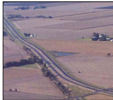
The IL-29 expressway alignment shifts to the east near Berry to avoid Illinois prairie grass.
