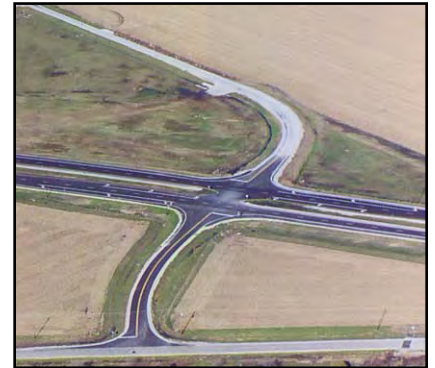
This relocated side road intersection near Berry was constructed at 90° to IL-29 to improve site distances.
